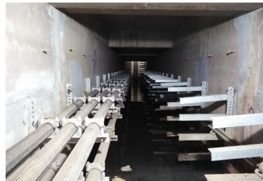
Fig.6. Square tunnel for the underground power cable installation
