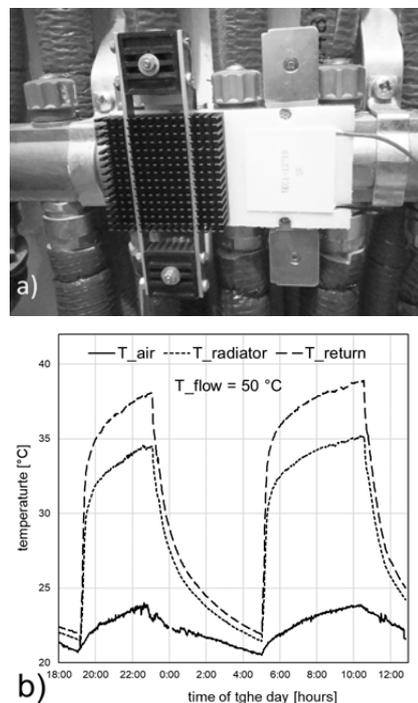
Fig. 6. Thermal energy harvester fitted to the return distributor of a domestic heating system: a) detailed view, b) exemplary temperature record on a winter day (detailed description in the text).
