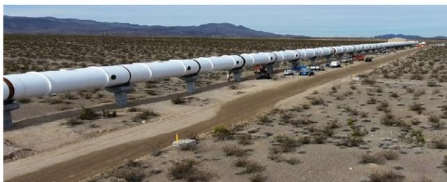
Fig. 9. Full-scale *Hyperloop* test track 488-m long in the Nevada desert built by *Virgin Hyperloop One* [7]
