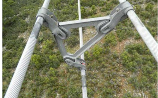
Fig. 3. Spacer damper for three cables [25].
