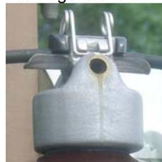
Fig. 1: Metal conductor clamp of covered conductor on which the analyses were performed.
