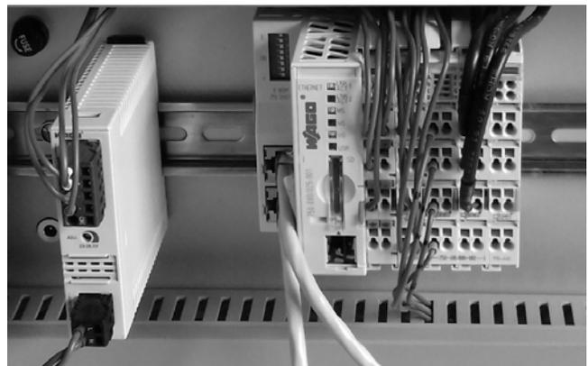
Fig. 2. WAGO I/O-SYSTEM 750 series PLC controller installed in the building switchboard
