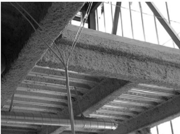
Fig.2. A floor made of steel deck plates (taken under construction)
