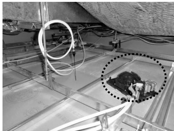
Fig.4. An antenna of a telemetry system (pole-type) and a LED socket (hatched circle) in the ceiling
