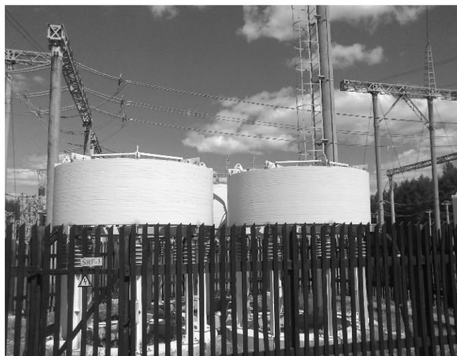
Fig 1. Shunt reactor
