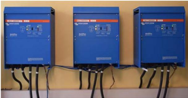
Fig. 1. View of three PV inverters type MultiPlus 48/5000/70
