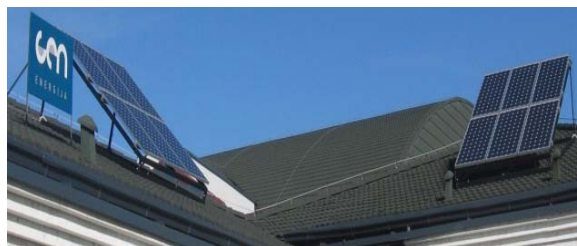
Fig. 1: From left to right: the fixed photovoltaic systems oriented to the east tilted 30° and the fixed photovoltaic systems oriented to the south tilted 30°.
