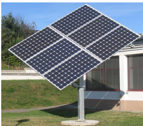
Fig. 2: The single axis photovoltaic tracking system tilted at 30°.
