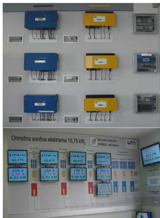
Fig. 4: Inverters and other operating devices in the control room and visual presentation of the photovoltaic systems.
