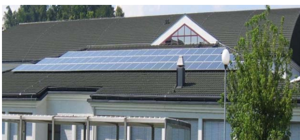
Fig. 3: The fixed photovoltaic system oriented to the south tilted at 15°.
