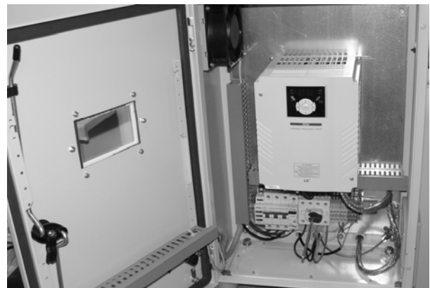
Fig.2. Motor power system with inverter LG iG5A
