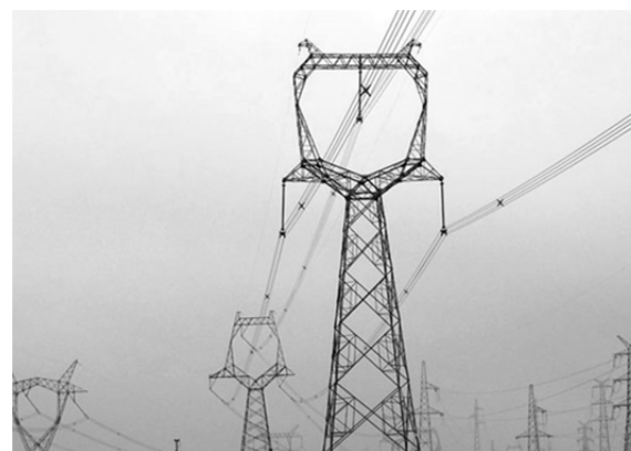
Rys.2. Linia 1000 kV Jindongnan-Jingmen [5]
