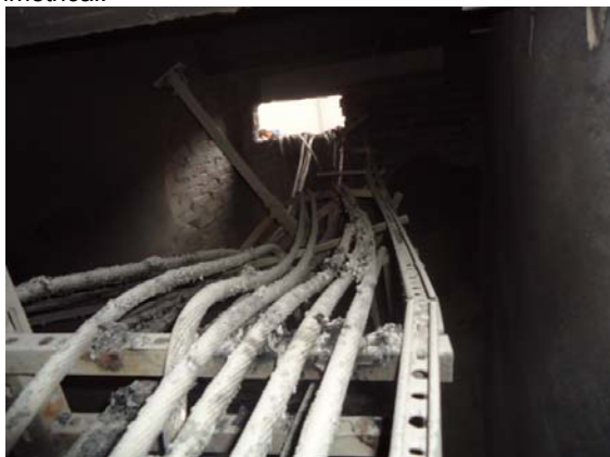
Fot.1 Cables after fault
