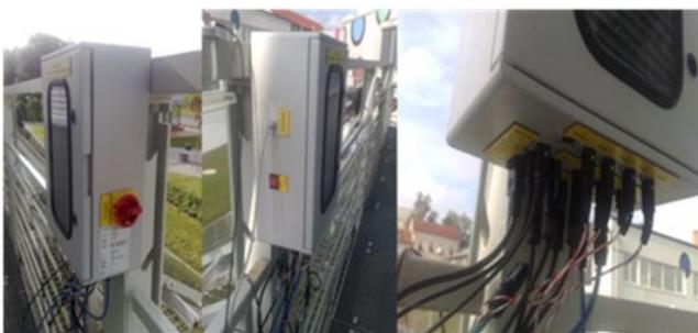
Fig.1. Measuring system for characteristics monitoring of PV modules (MSPV01)
