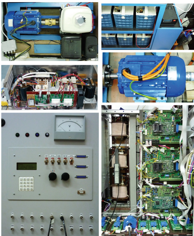
Fig. 6. Real photos of system components: (from top to bottom) combustion engine and PMSM generator, batteries, battery charger, PMSM vehicle drive motor, power electronics and control, front panel
