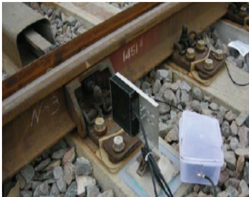
Fig. 8. Field installation of PSD laser displacement sensor
